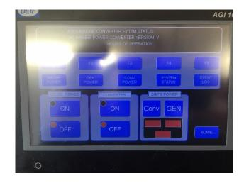
A customer had an issue with their remote shore power converter HMI screen used for transferring between shore and generator power. The screen did not power up correctly although 24vdc was present at the supply terminals. The screen was obsolete and replacing it with a modern equivalent would have additional cabling and also a larger screen which would lead to a new switchboard door and repositioning of instrumentation.
