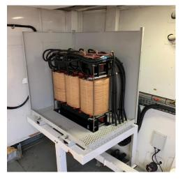
A customer had a problem wherby they could not operate their hotel services including air conditioning comfortably when moored due to an undersized shore power isolating transformer which had a rating of 152A full load current.
