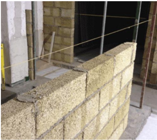
Interior Partition Wall made with GaiaBloc® & GaiaCast®
