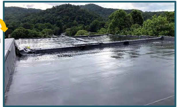
capped/ wrapped upright parapet wall
