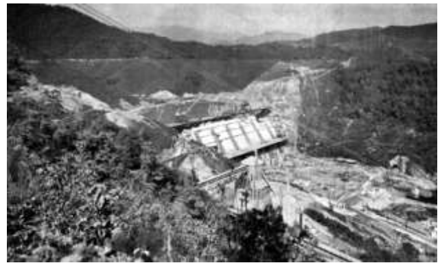
Fontana Dam under construction (www.grahamcounty.net)
