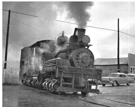
1926 Shay at Main and Depot Street, Robbinsville
