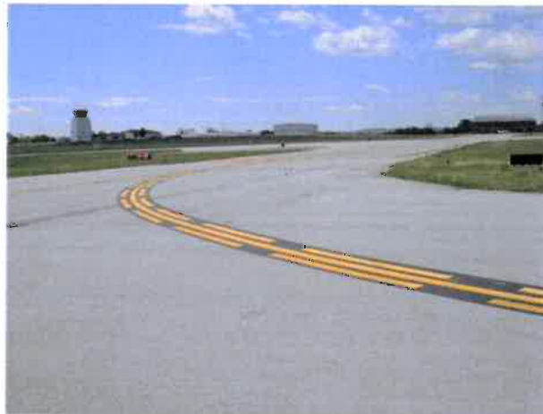
New enhance taxiway centerlines associated with runway hold lines located on Txy D at intersection of Txy C and Rwy 31
