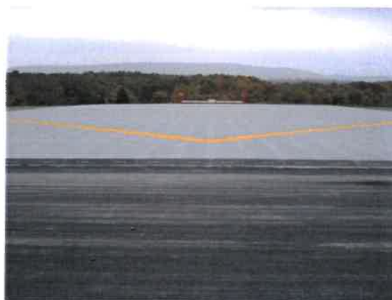
Chevron on EMAS bed at approach end of Rwy 31
