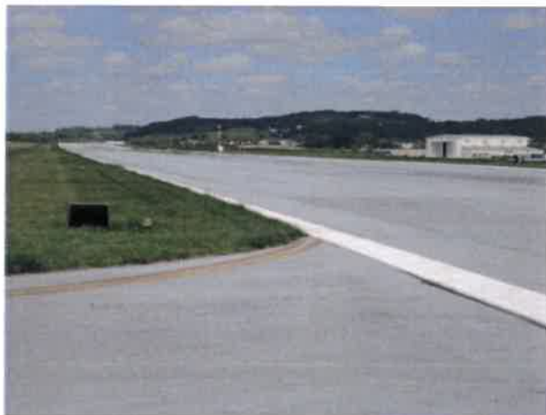
Runway edge lines locate on Rwy 31 at Txy D
