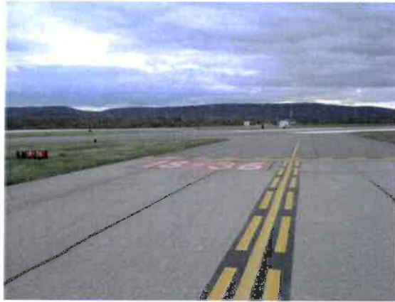
Surface painted hold sign on Txy B at Rwy 18/36
