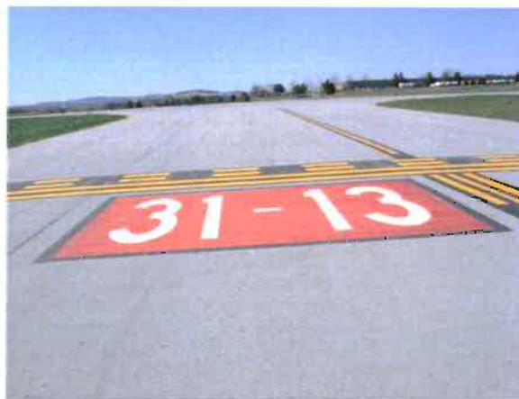
Surface painted hold sign on Txy F and Rwy 13/31
