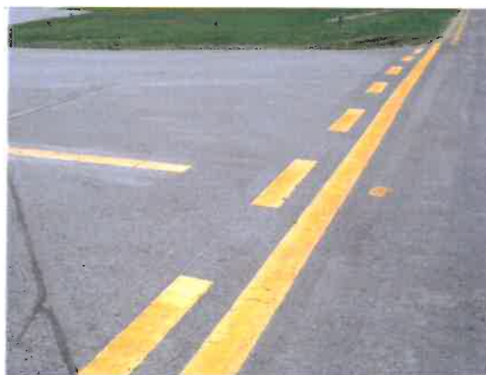
Non-Movement Area boundary line at East Apron and Txy A
