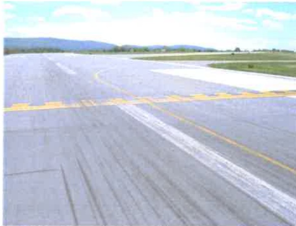
Runway 18/36 hold lines located on Rwy 13 at Txy J and Rwy 18/36 intersection. These would also be used as Rwy 13 "Land and Hold Short" lines for landing aircraft
