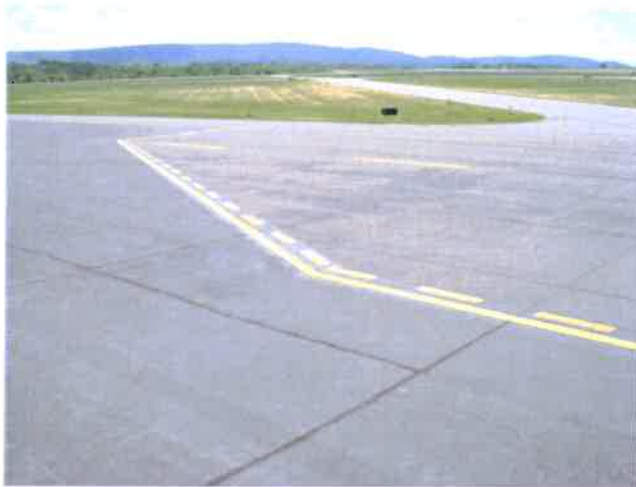
Non-Movement Area boundary line located on north apron at Txy G
