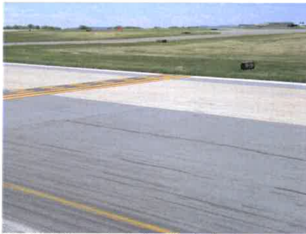
Rwy 18/36 hold line and associated hold sign located on Rwy 13
