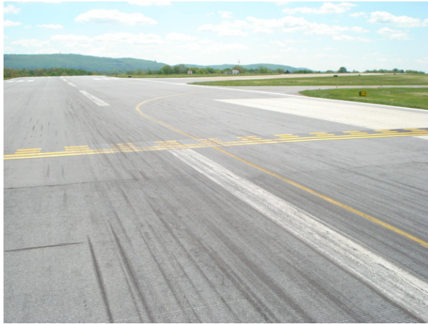
Runway 18/36 hold lines located on Rwy 13 at Txy J and Rwy 18/36 intersection. These would also be used as Rwy 13 “Land and Hold Short” lines for landing aircraft
