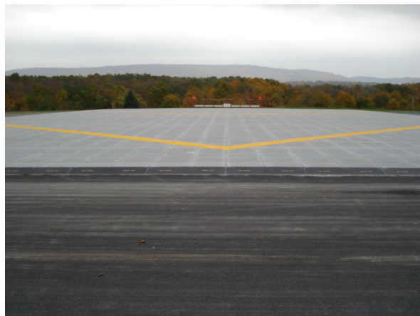
Chevron on EMAS bed at approach end of Rwy 31
