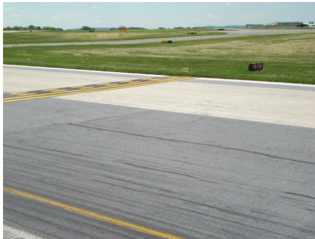
Rwy 18/36 hold line and associated hold sign located on Rwy 13
