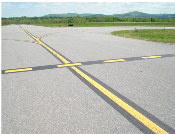
Taxiway intersection hold line located on Txy D at intersection of Txy G
