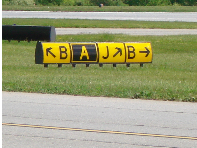
Taxiway directional sign located on Txy A
