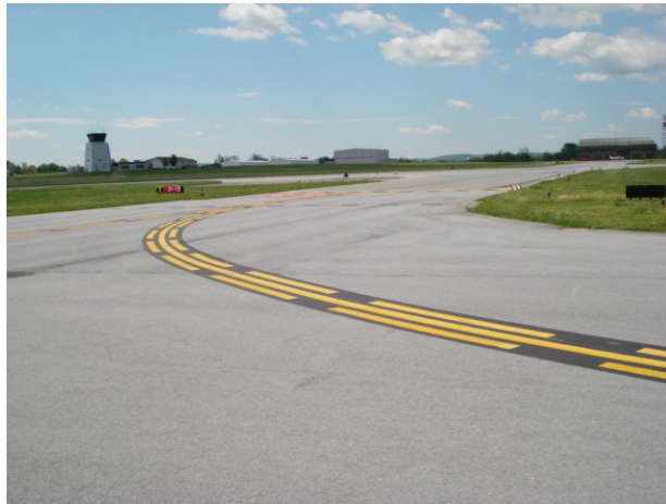
New enhance taxiway centerlines associated with runway hold lines located on Txy D at intersection of Txy C and Rwy 31
