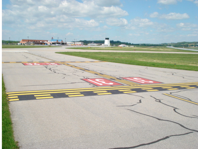
Double HOLD lines on Txy B between Rwy 31 and 36 Note: Make sure you are located at the proper hold line!
