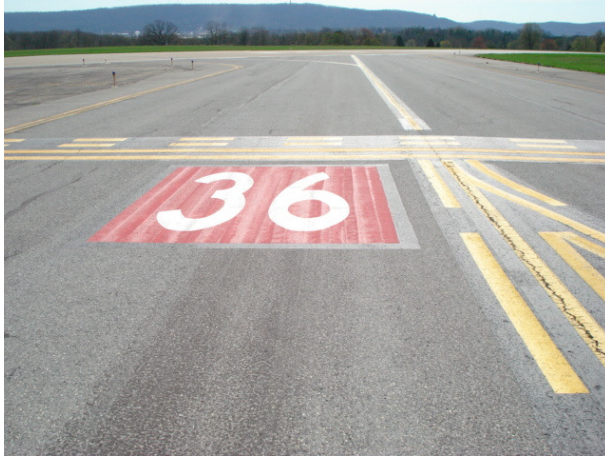
Surface painted hold sign on Txy A at Rwy 36 approach
