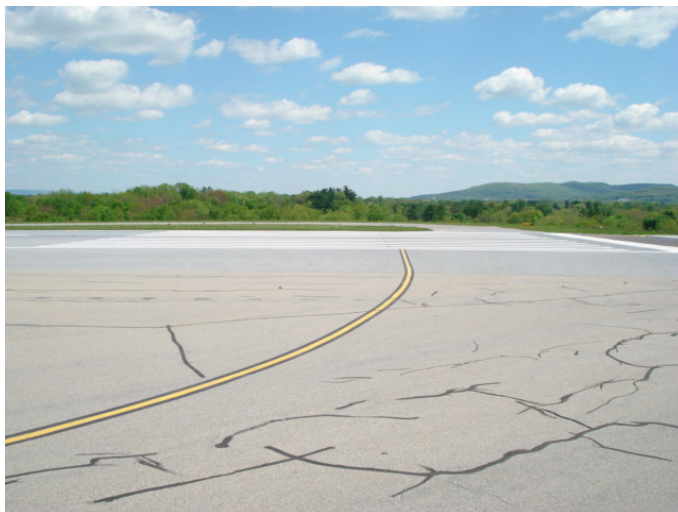
Taxiway lead-in line and Threshold bars located at Rwy 31 approach end
