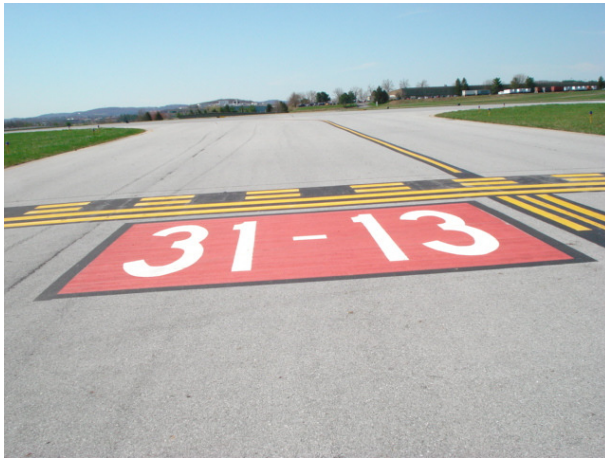
Surface painted hold sign on Txy F and Rwy 13/31
