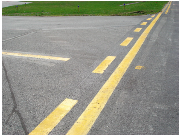
Non-Movement Area boundary line at East Apron and Txy A
