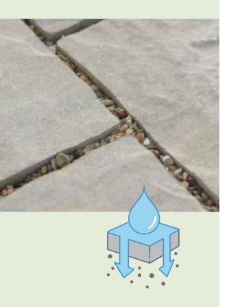
Permeable pavers look similar to traditional pavers but are designed with special spacer bars that create a wider joint.
