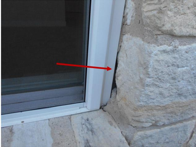
The seals for the side light windows at the front of the home were damaged and should be repaired.
