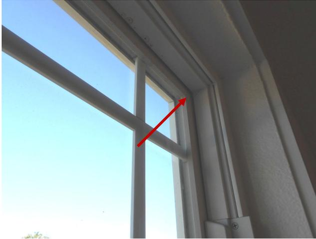
Safety glass etchings were not observed on the glass within the window in the master bathroom over the tub. This glass is required for windows close to the floor or in hazardous locations and is generally identified by an etching in the corner of the glass pane.
