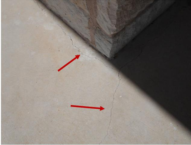
Minor cracking was observed in the foundation in the garage. This type of cracking is usually the result of shrinkage of the concrete as it cures. Shrinkage cracks are very common and should not be cause for alarm. This area of course, should be monitored.
