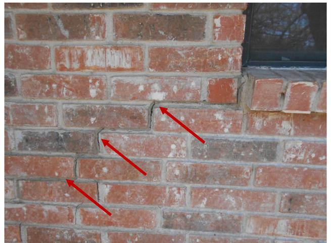
Slightly greater than typical foundation cracking was observed at the garage. The amount of movement does not suggest a serious structural problem. This area should, of course, be monitored. The rate of movement cannot be predicted during a one-time inspection.
