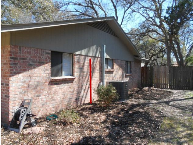
The area where the old refrigerant lines enter the home should be sealed to prevent water penetration.
