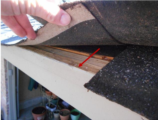
Tree branches should be trimmed away from the roofing material. This condition can lead to damaged roofing material and possible water penetration. Three to four feet of clearance is generally recommended.
