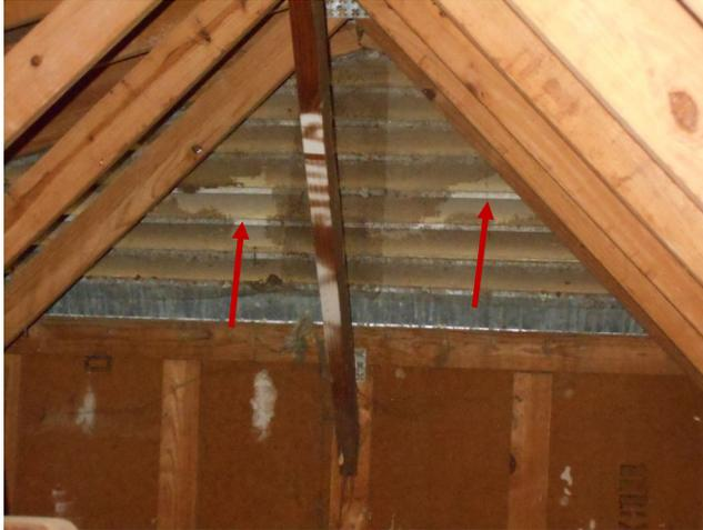
The current attic access hatch is considered to be a breach in the fire wall of the garage. By today's standards, a fire rated attic ladder, a hatch cover made of gypsum board or a separation wall between the garage attic and the residence attic is required.
