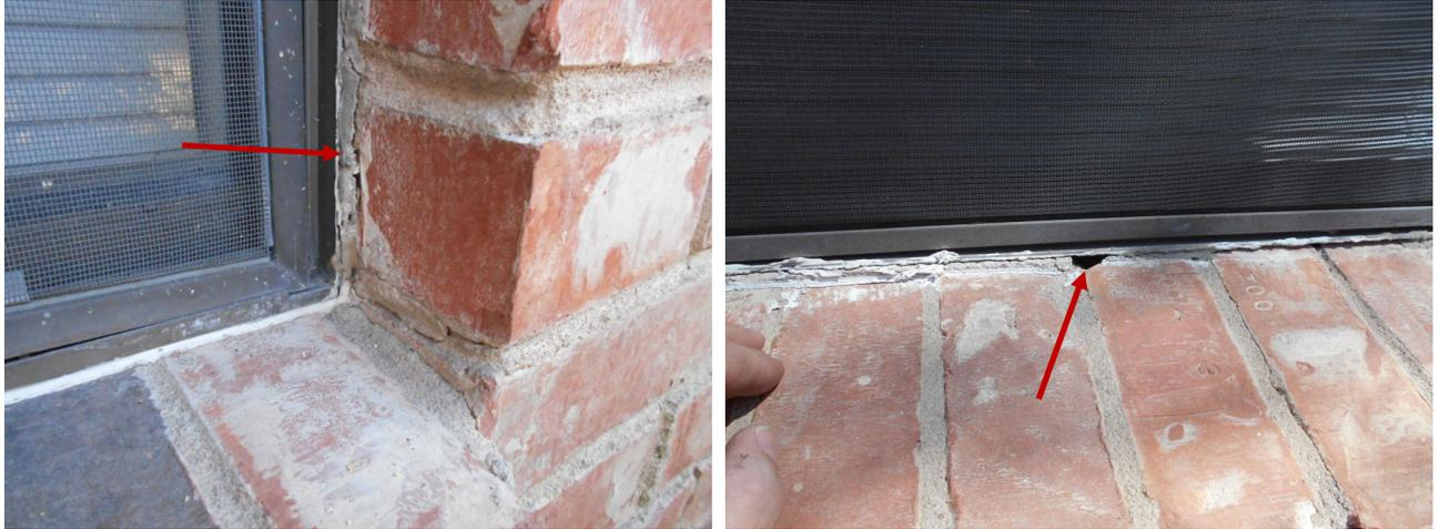
Damaged window glazing was observed in various locations. This is a minor defect and can be easily repaired.
