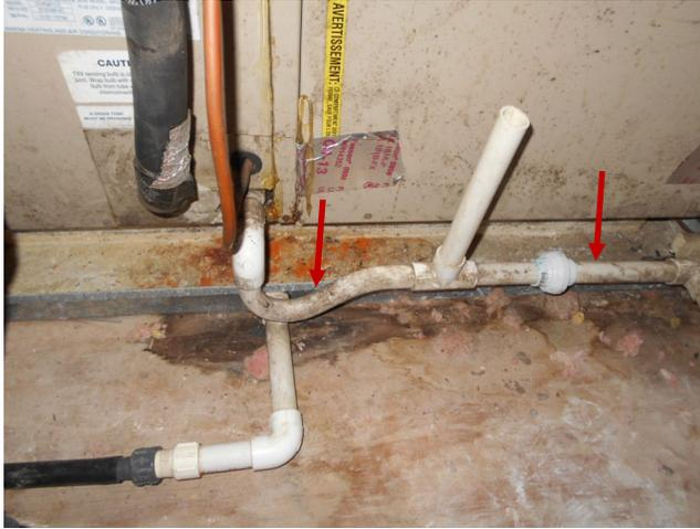
The condensate drain line for the air conditioner was observed to be open in the attic space. This line should be sealed to prevent water from spilling out and causing water damage to the ceiling.
