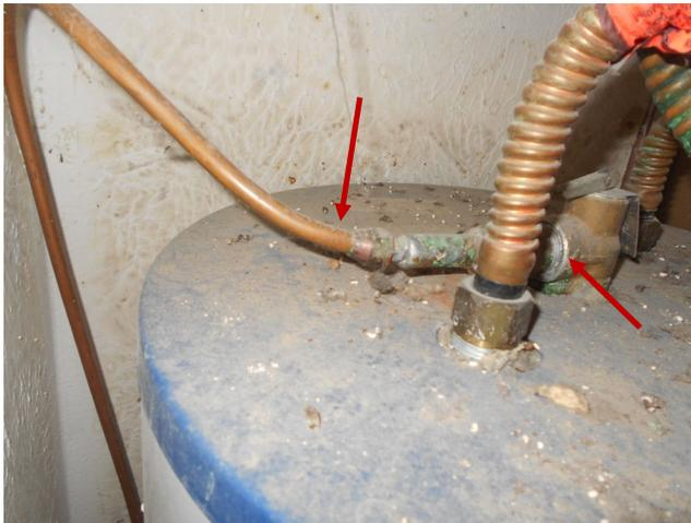
The drain line serving the T&P valve is not gravity feed; which is required under current building standards.
