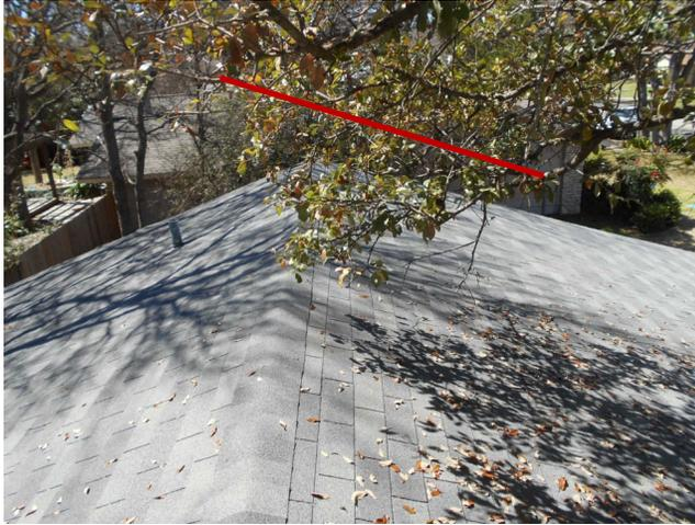
Debris should be removed from the roofing. This condition can trap moisture and shorten the life of the roofing materials.
