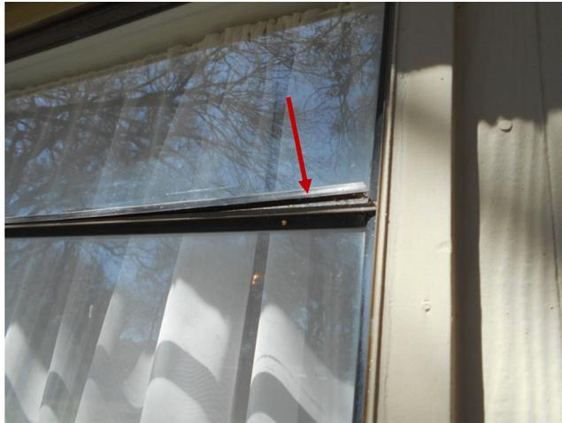
The spiral balancer for a window in the breakfast room is damaged. The spiral balancer keeps the window open.
