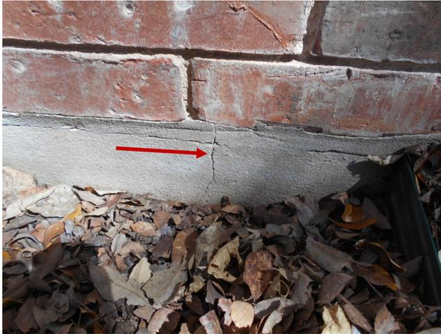
Cracks were observed on the exterior walls along the south side of the house. This implies that some structural movement of the building has occurred.
