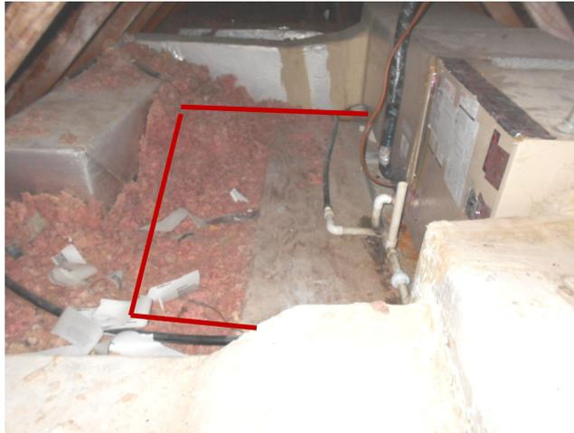
The door of the furnace is damaged and drawing air into the unit. This should be repaired.
