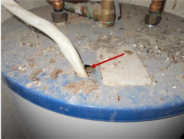
The T&P drain line is required to be the same size as the valve outlet. It is recommended that this be repaired for safety reasons.
