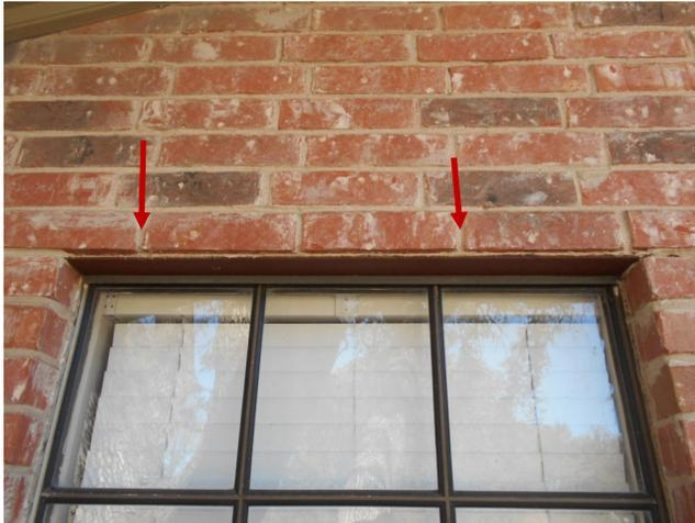
Pronounced exterior wall separation was observed at the front of the garage and kitchen window. This implies that structural movement of the building has occurred. The rate of movement cannot be predicted during a one-time inspection. A foundation company should be consulted to further evaluate this condition and the remedies available for correction.
