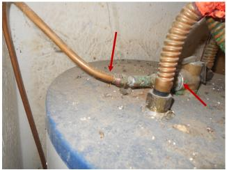
The drain line serving the T&P valve is not gravity feed; which is required under current building standards. The discharge piping serving the Temperature and Pressure Relief (TPR) Valve for the water heater should terminate not less than 6 inches or more than 24 inches above the floor. Repairs should be undertaken. Under current building standards, electric water heaters should be provided a means of service disconnect insight of the unit, which was not present at the time of inspection.
