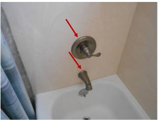
The static water pressure of the supply plumbing system exceeds 80 pounds per square inch (psi); it would be wise to install a pressure regulator. Otherwise, the plumbing system may be prone to leaks in piping, fittings or other equipment.
