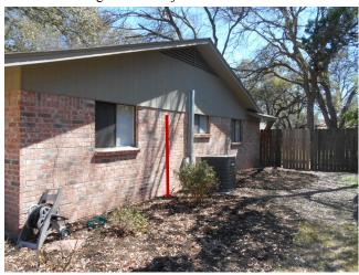
The area where the old refrigerant lines enter the home should be sealed to prevent water penetration.
