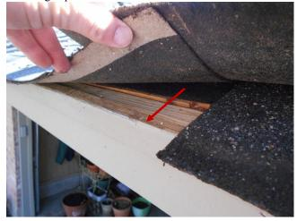
Tree branches should be trimmed away from the roofing material. This condition can lead to damaged roofing material and possible water penetration. Three to four feet of clearance in generally recommended.
