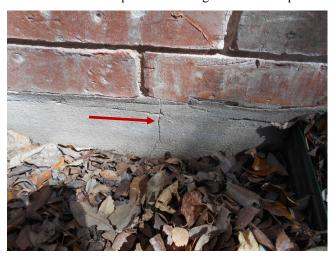
Cracks were observed on the exterior walls along the south side of the house. This implies that some structural movement of the building has occurred.
