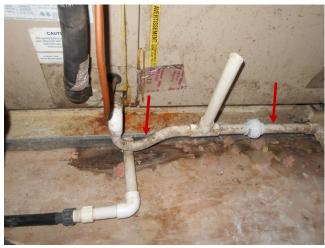
The condensate drain line for the air conditioner was observed to be open in the attic space. This line should be sealed to prevent water from spilling out and causing water damage to the ceiling.
