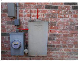
The exposed electrical conductors on the service mast should be protected. Repair by a licensed electrician is recommended.
