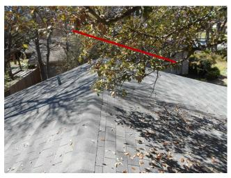
Debris should be removed from the roofing. This condition can trap moisture and shorten the life of the roofing materials.
