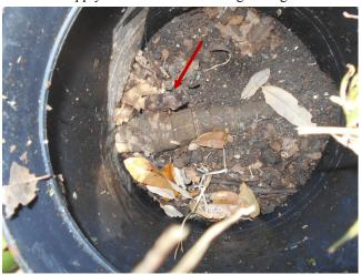
It is recommended that an anti-siphon device be added to all of the hose bib(s) to reduce the potential for potable water to contact a source of contamination. This condition should be repaired as is poses a potential health concern. This is a simple improvement and can be purchased at most hardware stores.
