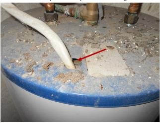
The T&P drain line is required to be the same size as the valve outlet. It is recommended that this be repaired for safety reasons.
