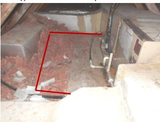
The door of the furnace is damaged and drawing air into the unit. This should be repaired.
