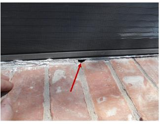
Damaged window glazing was observed in various locations. This is a minor defect and can be easily repaired.
