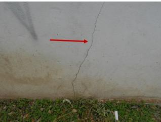
The soil line is too high at the front of the house. This condition can promote water and insect infiltration. Under today's building standards, there should be at least four (4) inches of foundation visible below masonry veneer and six (6) inches of foundation visible below wood veneer.
