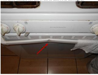
The range anti-tip prevention devices are not present and/or do not properly function providing a hazardous condition. Children are prone to use range and/or oven door as a step stool, which can tip the range resulting in a serious injury. This improvement is simple and the clip can be purchased at most hardware stores.
