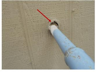
Deteriorated siding was observed in various locations. This item will need repair to prevent damage to the structure.
