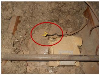
Improper electrical connections for the food waste disposer in unit D should be improved. All electrical connections should be made inside junction boxes fitted with cover plates.
