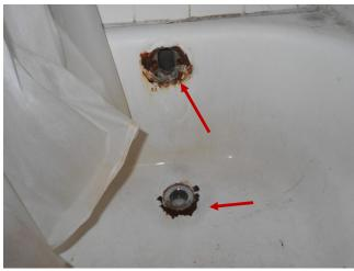
A supply valve handle in the bathroom of unit D is missing and should be replaced.
