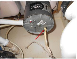
By today's standards the wiring leading to the food waste disposer should be a flexible plug in type or protected by conduit.
