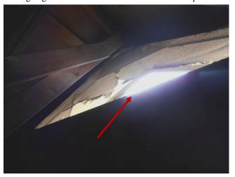
Substantial evidence of roof leakage was observed. This condition should be investigated further and repairs made, as necessary.
