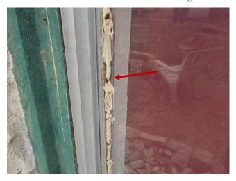
Flashing was missing above door and window trims that project from the wall. Flashing should be installed on top of the trim board and behind the wall covering. At a minimum improvement, a quality bead of caulking should be applied to the top trim boards to prevent water penetration.
