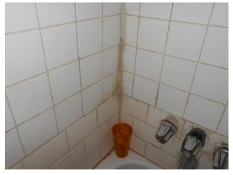
The supply valve covers and faucets for the showers should be sealed to the tile enclosures.
