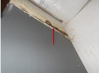
There is air leaking from a supply air plenum in the attic. This improvement is a minor repair and will reduce energy costs.
