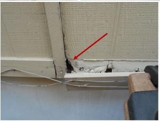
Deteriorated trim boards were observed in many locations. This item will need repair to prevent damage to the structure.
