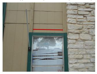
Window trims on the exterior of the house are in need of re-caulking to avoid water penetration.
