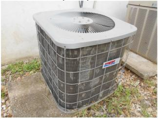
The outdoor units of the air conditioning system for units A and C are out of level. This should be improved.
