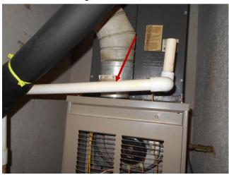
The air conditioning units should be provided with auxiliary drains or a device that will shut off the units in the event the primary drain lines become obstructed.
