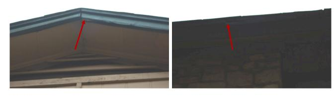
Damaged gable and roof vent screens should be repaired as needed to prevent vermin entry into the attic space.
