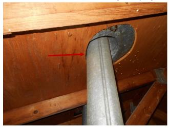
The duct insulation covering in the attic is damaged and pulling loose. Repair or replacement will be needed. An HVAC company should be consulted.
