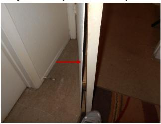
The door in many locations should be trimmed or adjusted as necessary to work properly. Missing door hardware to the furnace closet in unit B should be replaced. Damaged or non-functional door hardware in various locations should be repaired. Improperly sized doors were observed in various locations.
