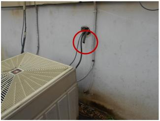
Damaged insulation on refrigerant lines should be repaired. This will help with the efficiency of the systems.
