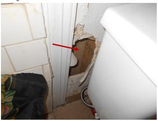
Water damage and moisture was noted in the living room wall of unit B. The cause for the damage should be determined and repairs undertaken, if necessary, to prevent structural damage.
