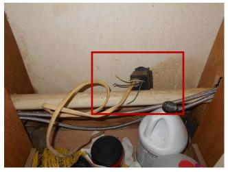
Outlets are damaged in the west bedroom of unit C. They should be replaced.
