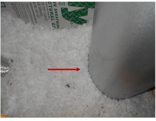
Fire stopping in the attic surrounding the chimney flue is not properly installed. *This should be corrected as this poses a fire hazard*.
