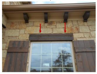
The header over the window at the front of the home should be sealed to prevent water penetration.
