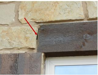
Openings in the mortar joints along the south side of the house should be sealed as necessary to prevent water penetration.
