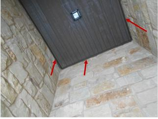
There was an insufficient amount of weep holes found at the foundation level at the front entrance. Weep holes allow moisture to drain from the wall cavity due to penetration or condensation. Drilling weep holes post construction is routine and simple. This is a common observation.
