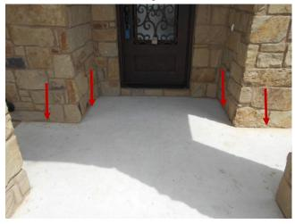
There was an insufficient amount of weep holes found above the lintels at the front of the home. Weep holes allow moisture to drain from the wall cavity due to penetration or condensation. Drilling weep holes post construction is routine and simple. This is a common observation.
