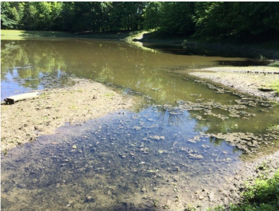
View of of large amount of sediment accumulation at the southern edge of the basin.
