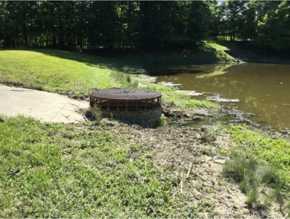
View of outlet structure for the basin.
