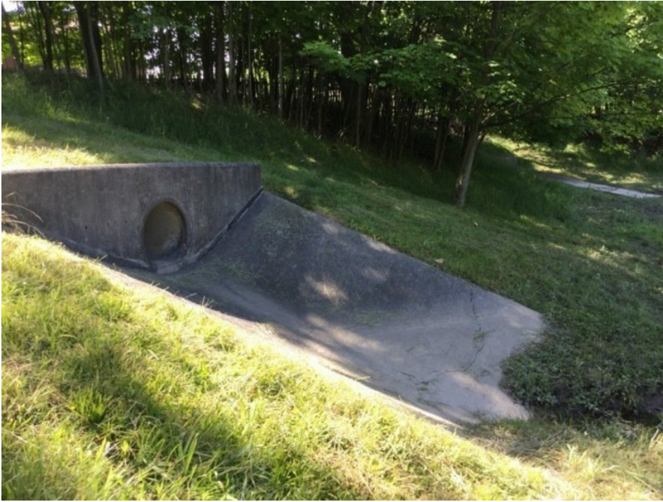
View of inflow structure along the eastern edge of the basin.
