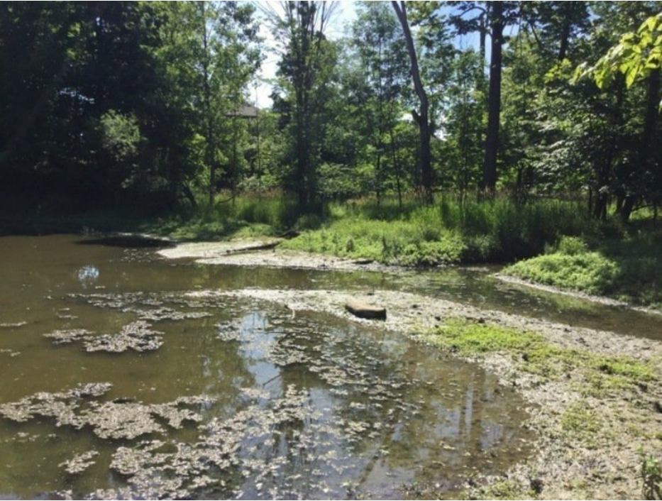
View of two inflow paths along the southern edge of the basin with large amount of sediment accumulation at the inflow.
