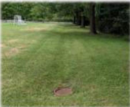
Circular Basin 1 (CB1) looking west within the drainage swale of Heasley Soccer Fields
