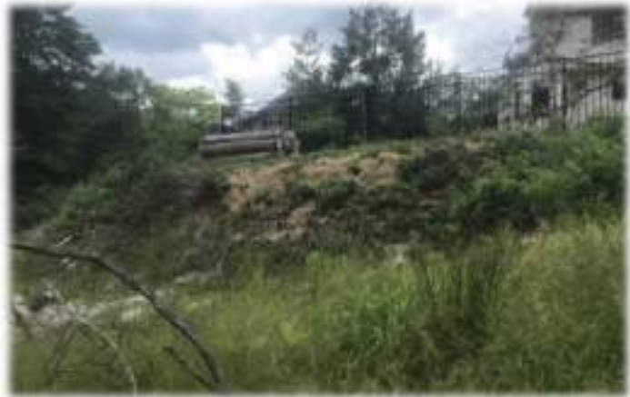
Yard waste/debris within Common Area PPN 489-21-035
