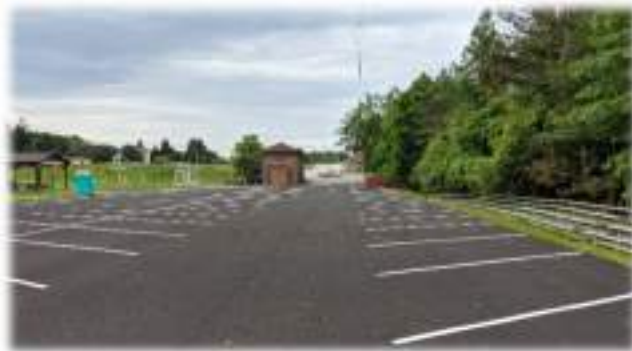
Looking south, view of parking lot draining north towards single inlet basin.
