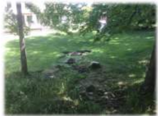
Figure 2. Drainage channel to basins at 5030 Corkwood
