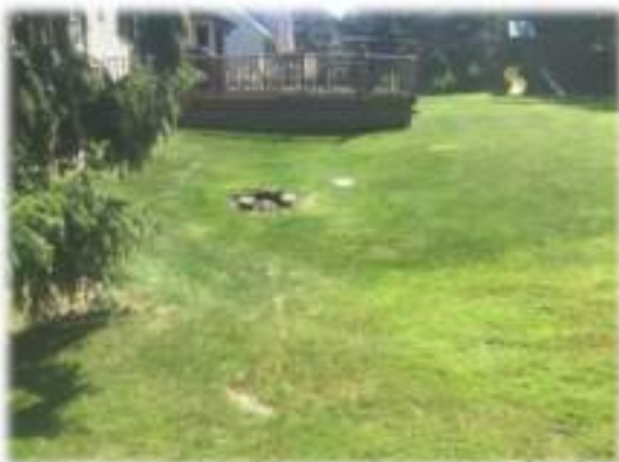
Figure 3. Downstream beehive basin at 5030 Corkwood Drive
