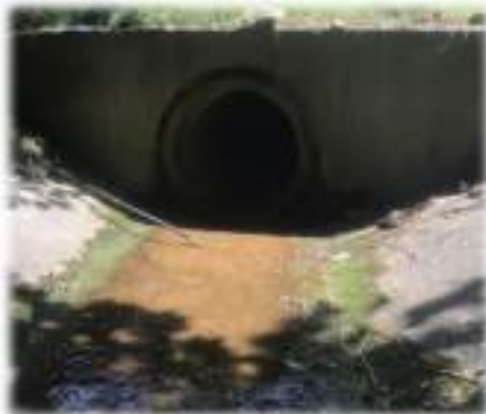
5031 Corkwood Drive outfall
