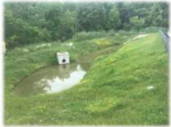
Stormwater basin west of church parking expansion.
