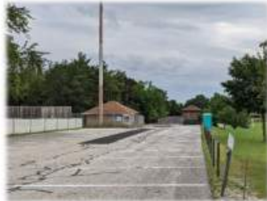
Southern portion of parking lot. No inlet basins.
