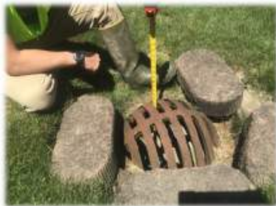
Figure 4. Downstream beehive basin at 5030 Corkwood Drive
