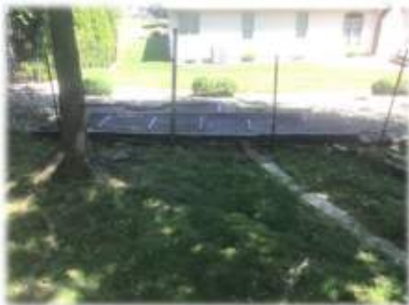
Figure 5. Screening over inlet basin at 5060 Corkwood Drive
