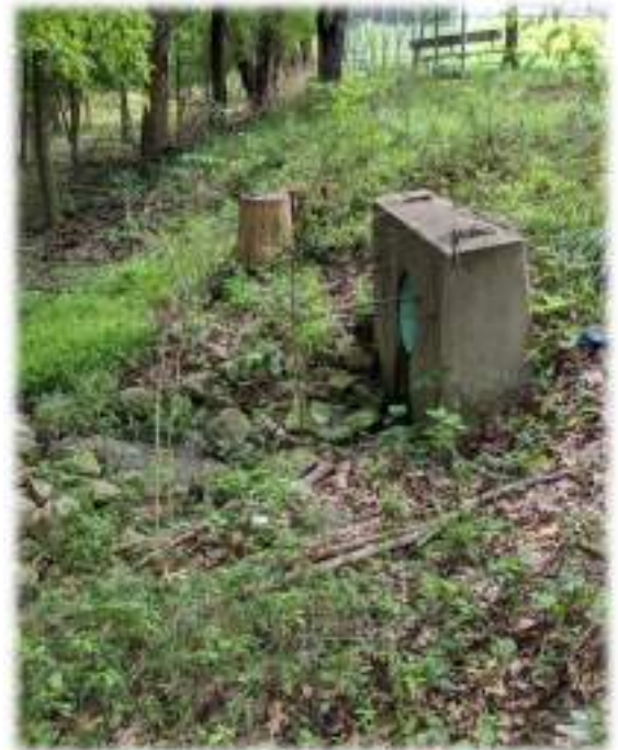
View looking south at HW-1 (see aerial view (left) for location) which discharges the storm drains along the northern field border.
