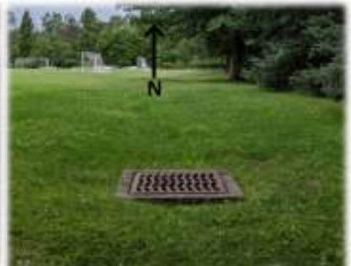
Inlet Basin 3 (IB3) looking west within drainage swale of Heasley Soccer Fields
