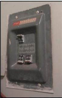
**Electrical Panel:** Make sure it's in working order, at least 100 amps (unless it's in a small apartment), and not a Federal Pacific or Pushmatic panel, both of which you should probably replace.
