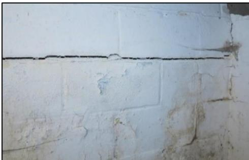
**Foundation Movement:** Anything over four inches should probably be braced or have “dead men” added. Much more than that and the wall might need to be pushed back, which is very expensive. (Pro tip: If you can’t tell how much the wall has moved, go outside and run your finger along the bottom of the siding. It should go about to your knuckle. But just running it along the foundation wall should give you an idea of where and how much the wall has moved.)
