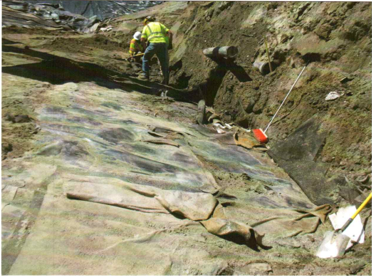
Figure 2 Existing Landfill Construction Damage
