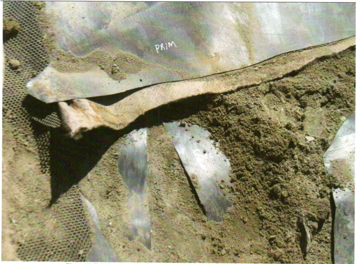
Figure 1 Existing Landfill Equipment Damage below Proposed Tie-in Seam.
