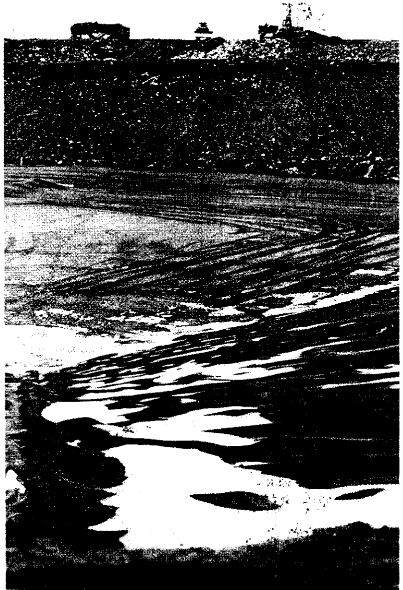
READY TO BE FILLED-- The fourth and final double-lined cell of the Consumat Sanco landfill expansion area sits ready to accept refuse by year's end. In the background is the No. 3 cell of the expansion area, where trash is currently being deposited.
