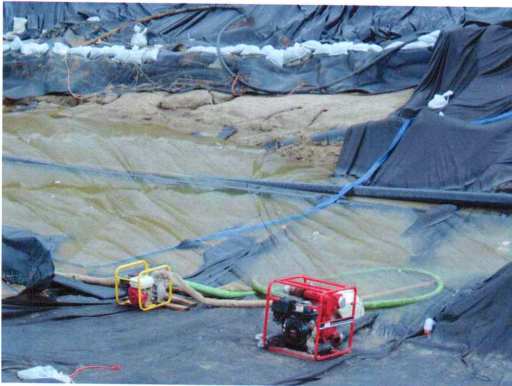
Contaminated storm water in Phase II Stage II sump being pumped.
