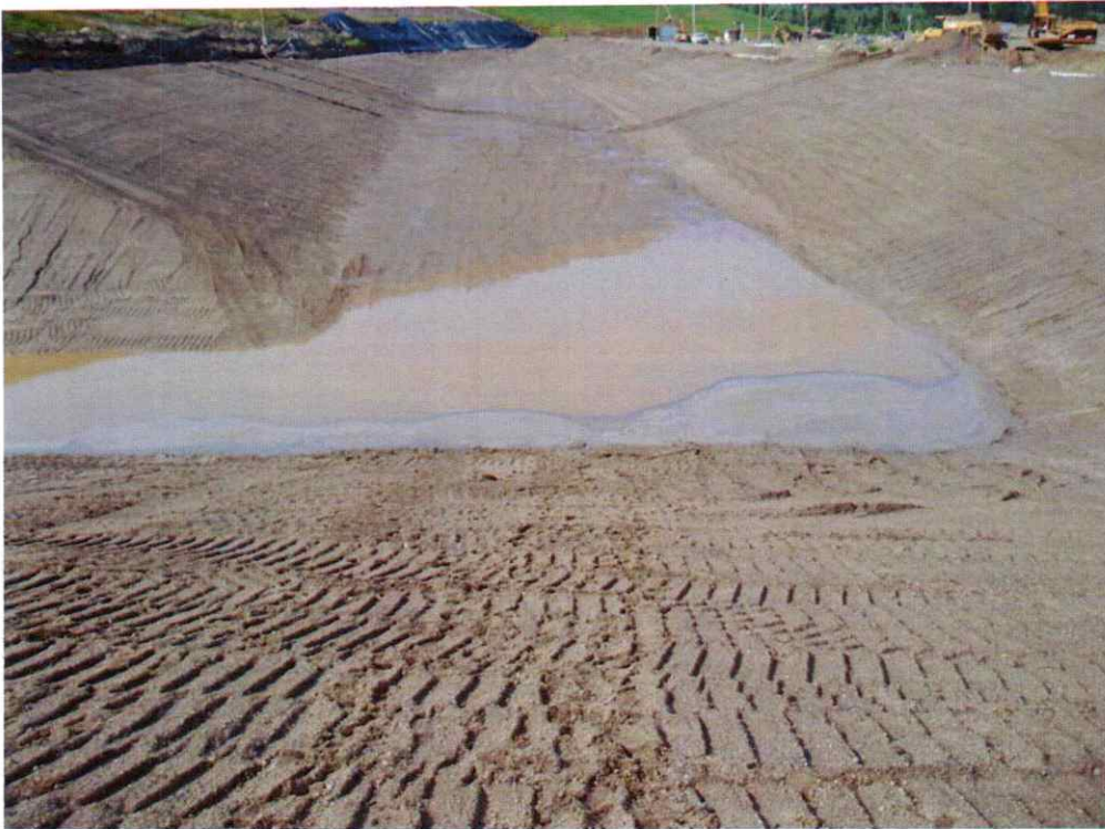
Contaminated storm water in Phase IV Stage I sump.
