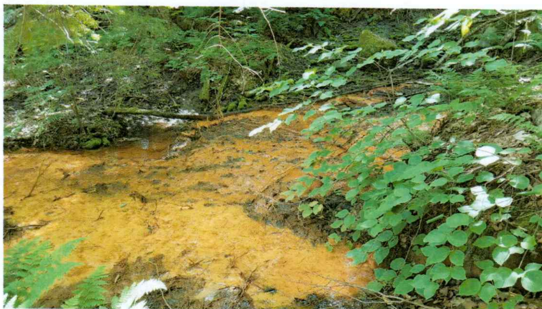
Photo 6. BHW1 upslope portion where iron staining and groundwater seepage is most prevalent (F23) (6/23/23)
