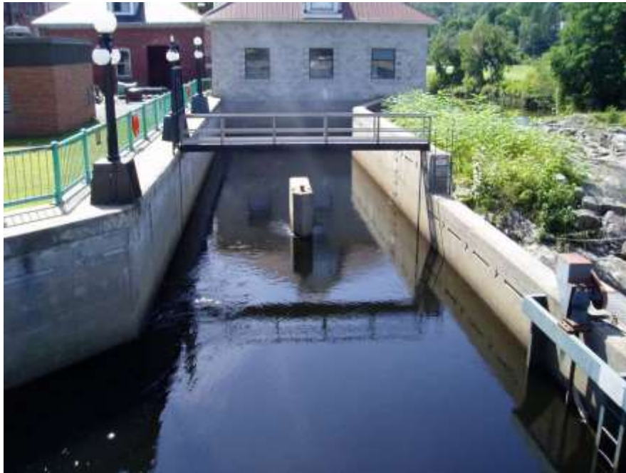
Lisbon Dam Powerhouse and canal Photo by Field Geology Services, 2009
