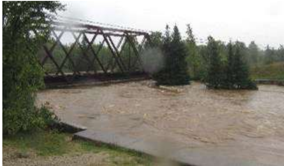
Tropical Storm Irene floodwaters carrying silt Photo by Leslie Bergum, 2011
