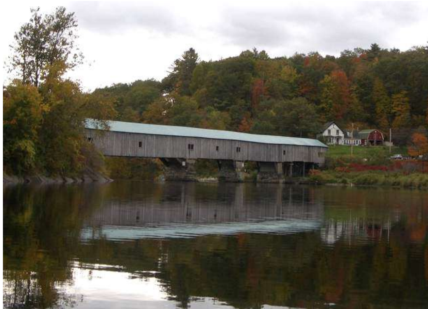
Bath Covered Bridge, Photo by Field Geology Services, 2009
