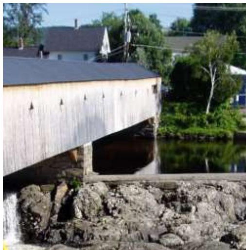
Haverhill-Bath Covered Bridge Photo by Field Geology Services, 2009
