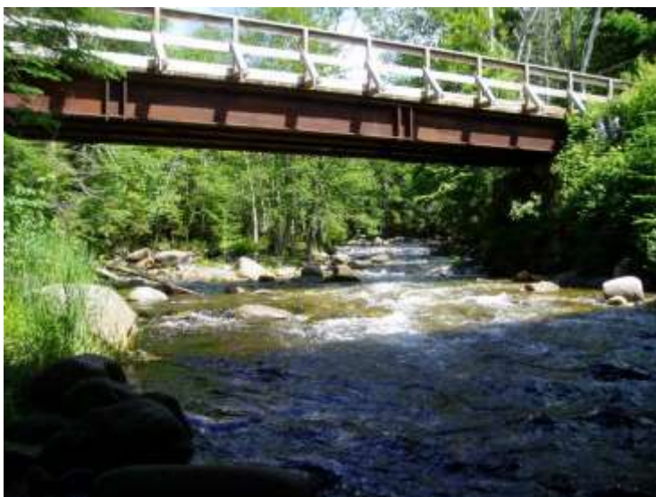
Snowmobile bridge over the Ammonoosuc River Photo by Field Geology Services, 2009
