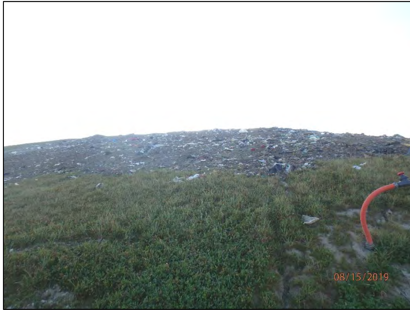
P8150024: Working face in the western portion of Stage V/Phase II, as viewed from the west and looking upslope in an easterly direction.
