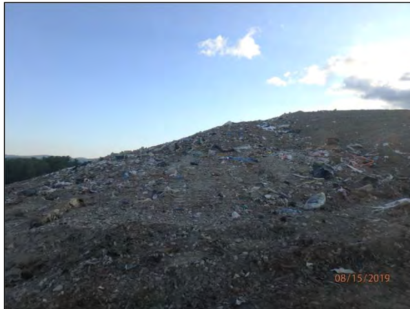
P8150021: Working face located in the western portion of Stage V/Phase II, as viewed from the south and looking in a northerly direction.
