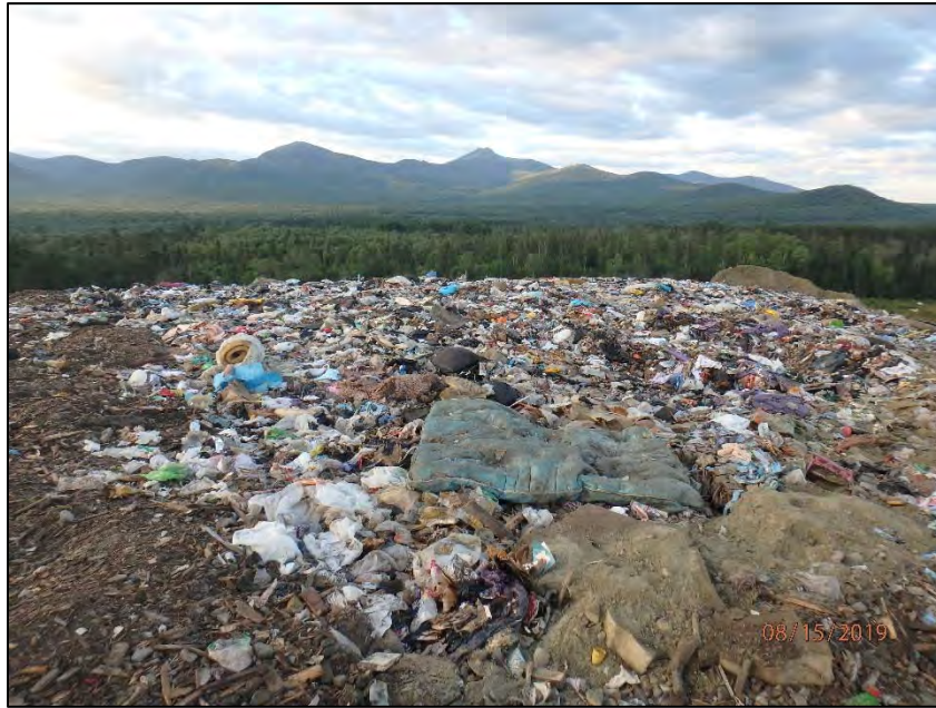
P8150019: Working face in the southern portion of Stage IV/Phase II following the removal of the daily cover tarps, as viewed from the north and looking in a southwesterly direction.
