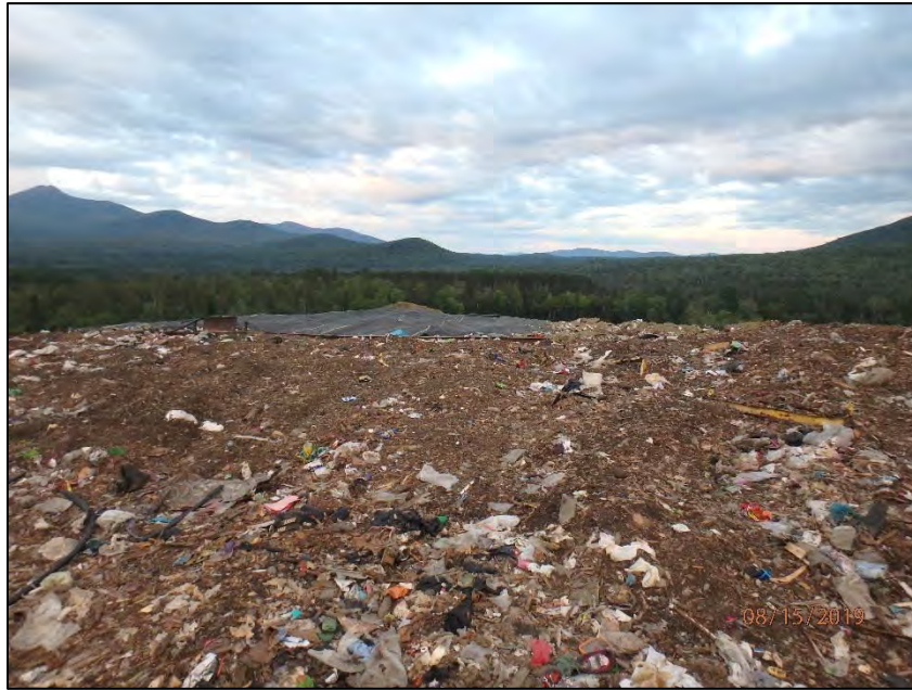
P8150001: Overview of the southern portion of Stage IV/Phase II, prior to the working face being uncovered. Looking west. The tarps present in the center of the photograph are the approximate location of a working face.
