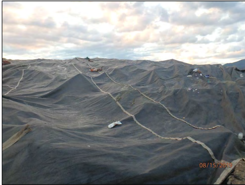
P8150007: Representative photograph of the tarp used as daily cover in the southern portion of Stage IV/Phase II, as viewed from the west and looking upslope in an easterly direction.
