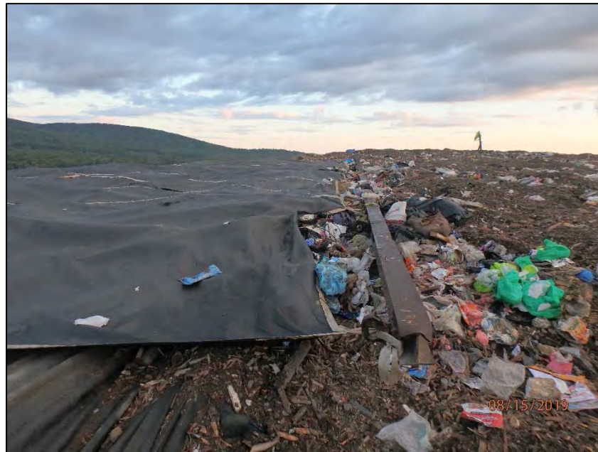
P8150004: Working face in the southern portion of Stage IV/Phase II, prior to the working face being uncovered. Looking north.
