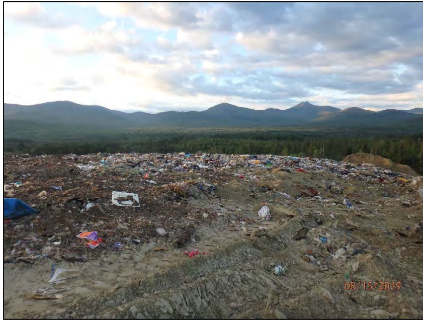
P8150017: Overview of the working face in the southern portion of Stage IV/Phase II following the removal of the daily cover tarps, as viewed from the north and looking in a southerly direction.
