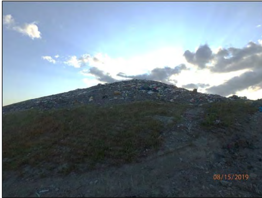
P8150022: Overview of the working face in the western portion of Stage V/Phase II, as viewed from the west and looking in an easterly direction.
