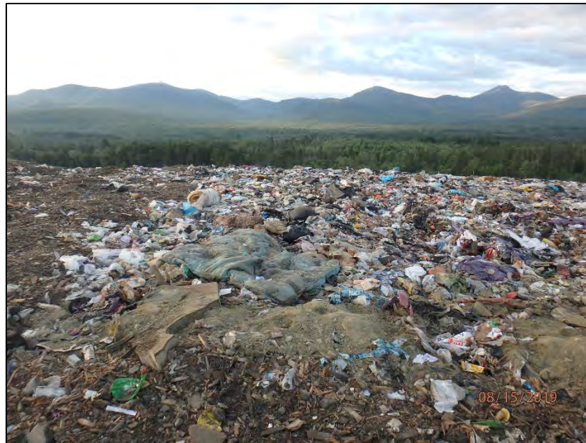
P8150018: Working face in the southern portion of Stage IV/Phase II following the removal of the daily cover tarps, as viewed from the north and looking in a southerly direction.
