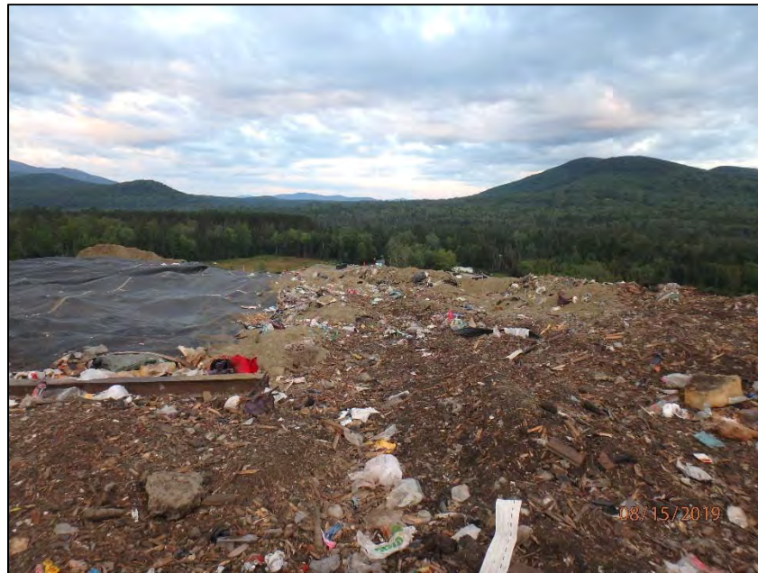
P8150002: Working face in the southern portion of Stage IV/Phase II, prior to the working face being uncovered. Looking west. Exposed waste is visible along the northern edge of the daily cover tarp.
