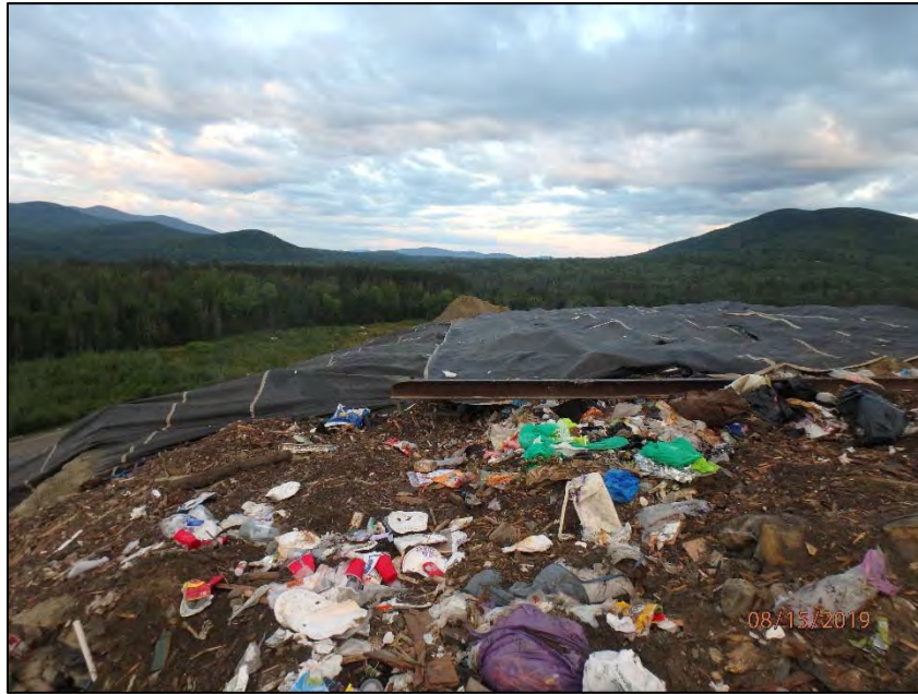
P8150003: Working face in the southern portion of Stage IV/Phase II, prior to the working face being uncovered. Looking west.
