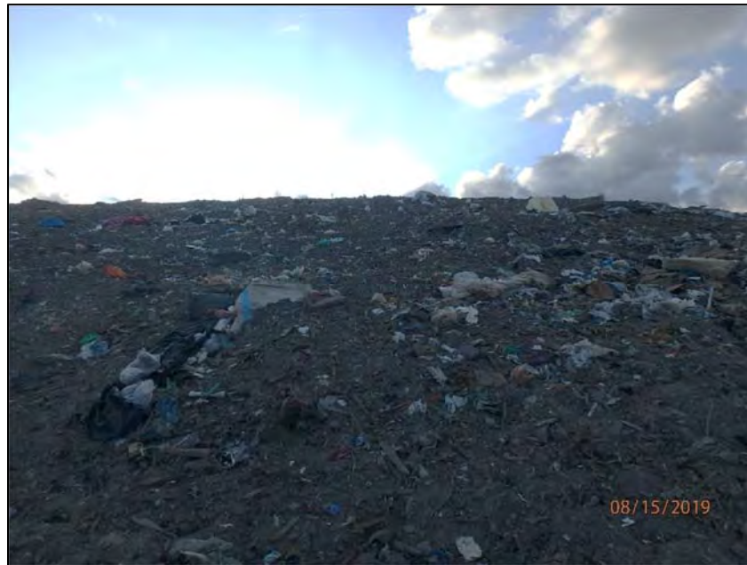
P8150023: Working face located in the western portion of Stage V/Phase II, as viewed from the west and looking upslope in an easterly direction.
