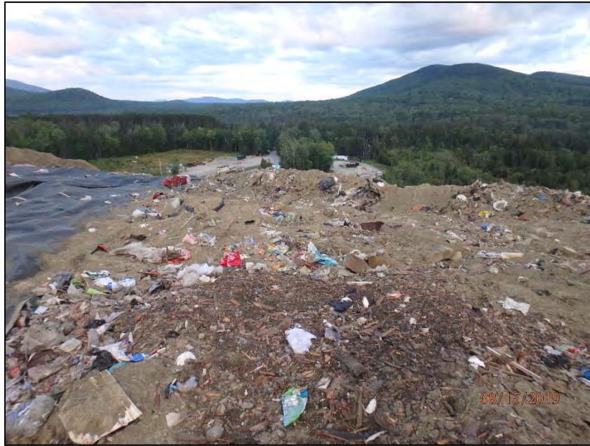
P8150005: Southern portion of Stage IV/Phase II, prior to the working face being uncovered. Looking west. Exposed waste is visible beyond the northern edge of the tarp.
