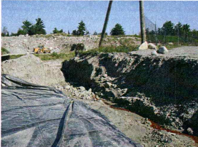
Picture 4. This picture is looking north towards MW 913M. The open trench is where the 36" culvert connecting the Stage 1 Phase 1 down chute to detention pond 3 was located.
