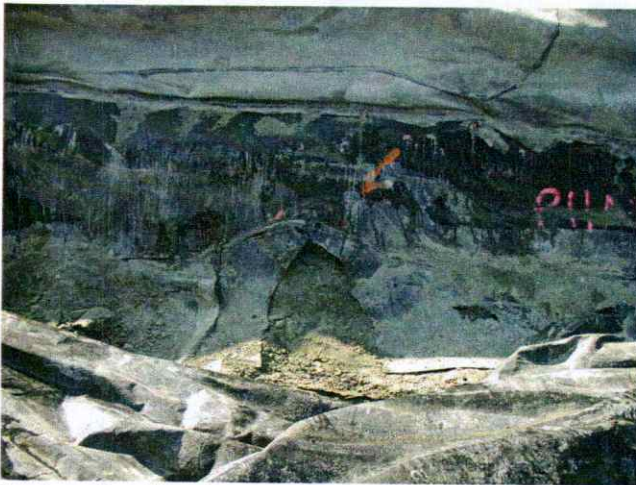
Picture 3. This picture is looking north at the Stage 1 Phase 1 anchor trench. Note arrow pointing out hole in geomembrane cap.
