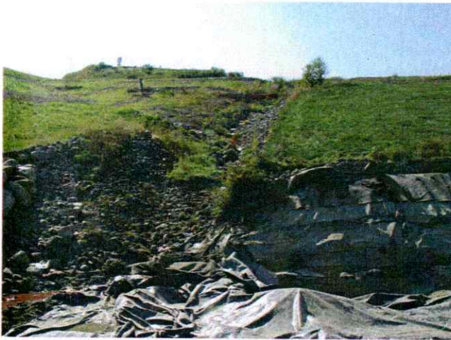
Picture 2. This picture is looking up (south) the Stage 1 Phase 1 downchute. The excavated anchor trench is to the right.
