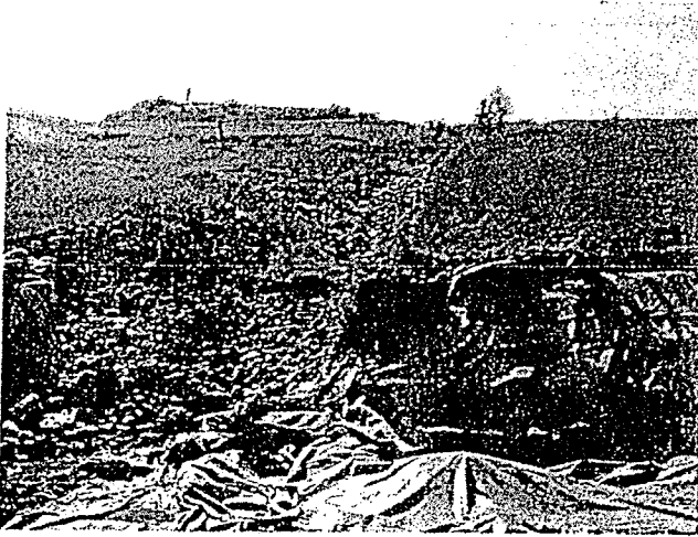
Picture 2. This picture is looking up (south) the Stage 1 Phase 1 downchute. The excavated anchor trench is to the right.
