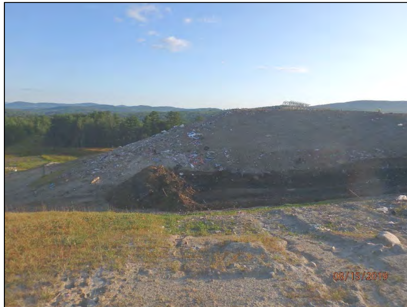
P8150025: Working face in the western portion of Stage V/Phase II, as viewed from the south. Prior to this photograph, NCES personnel removed a limited layer of cover material on the southern edge of the Stage V/Phase II working face to create room in which to deposit a load of sludge.
