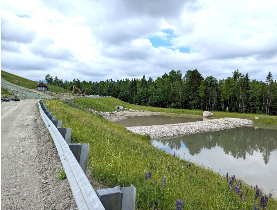
PXL_20240612_150436038: Stormwater Pond near Stage V, sediment observed in forebay
