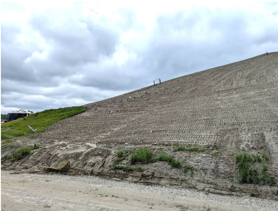
PXL_20240612_151157977: Cap 4 area with waste visible where gas header pipe was excavated and re-pitched
