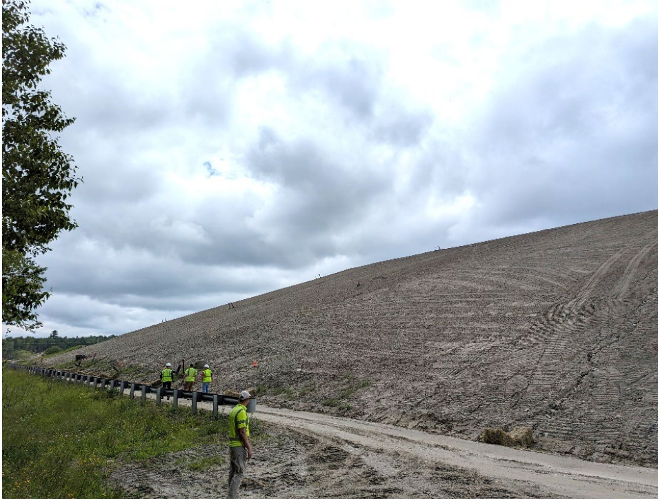
PXL_20240612_150815453: Cap 4 area with intermediate cover
