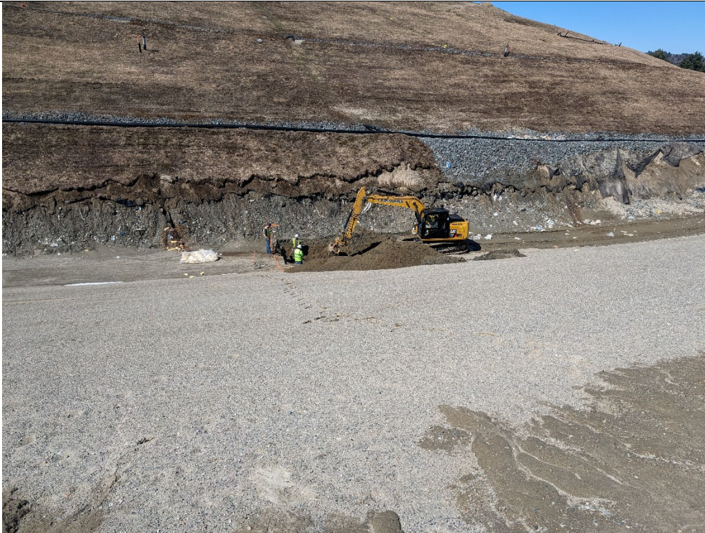
Excavating from south to north
