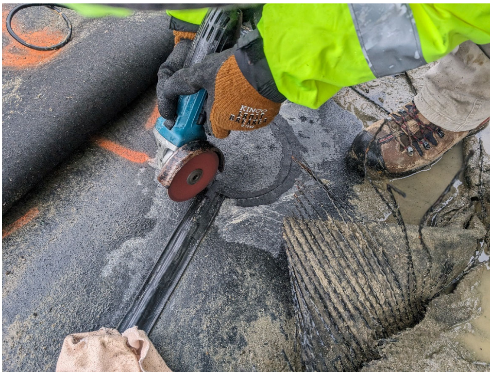
Patch being prepared for extrusion welding.
