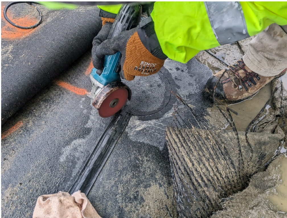
Patch being prepared for extrusion welding.
