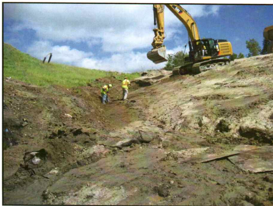
Uncovering Anchor Trench – Looking Southeast
