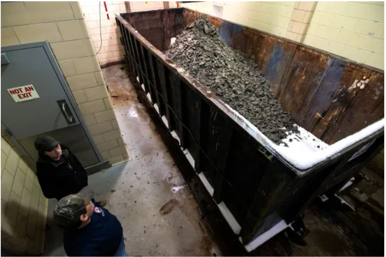
Amanda Smith and Phil Besse stand next to a 30-yard container as it fills with biosolids at the City of Bangor Wastewater Treatment Plant on Main Street. According to Smith, three 30-yard containers of biosolids are produced every day at the plant. Two of those three containers are now being shipped to Canada. Credit: Linda Coan O'Kresik / BDN
