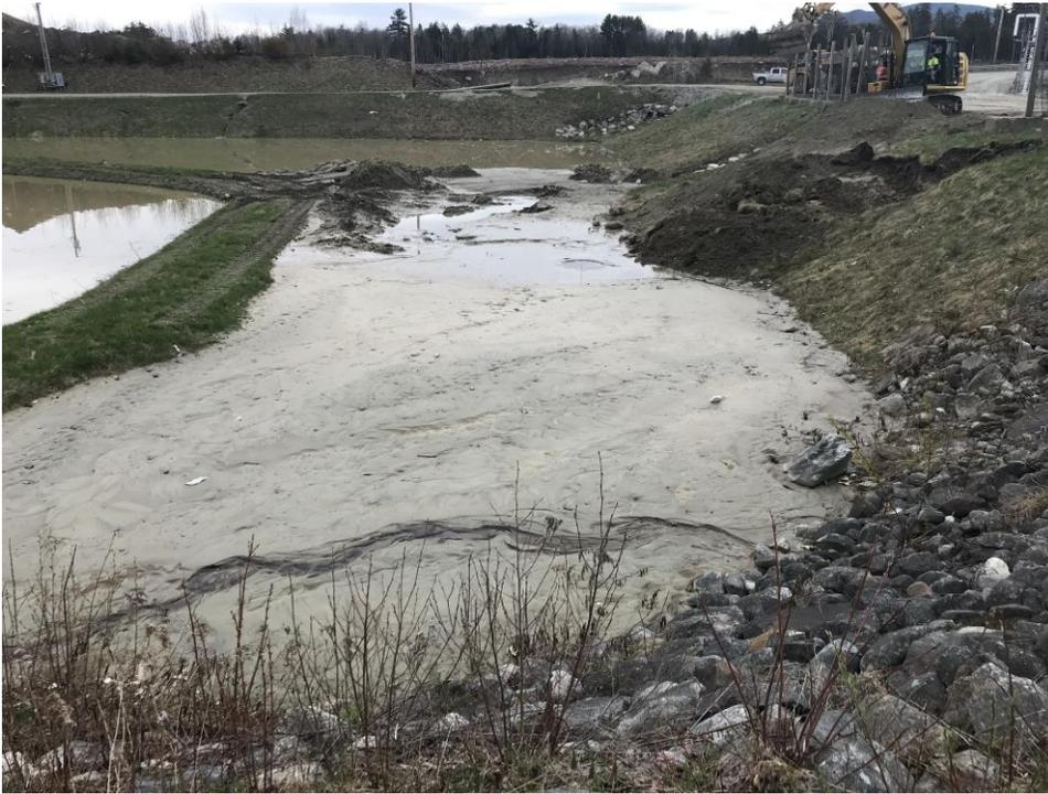
Sediment and leachate in retention basin, note the construction of the ramp to the right of the photo.
