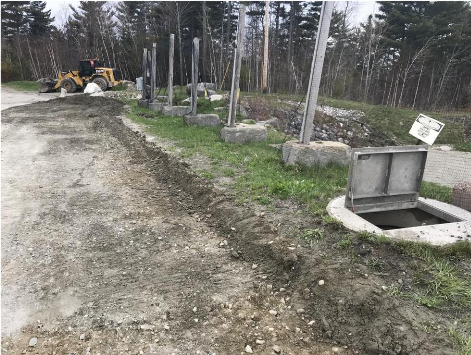
Overland route leachate followed to the retention pond. Contaminated soil was scraped and removed. Drainage ditch leading into the pond is behind the loader in the photo. Manhole where the release originated is behind and to the left of the viewer.
