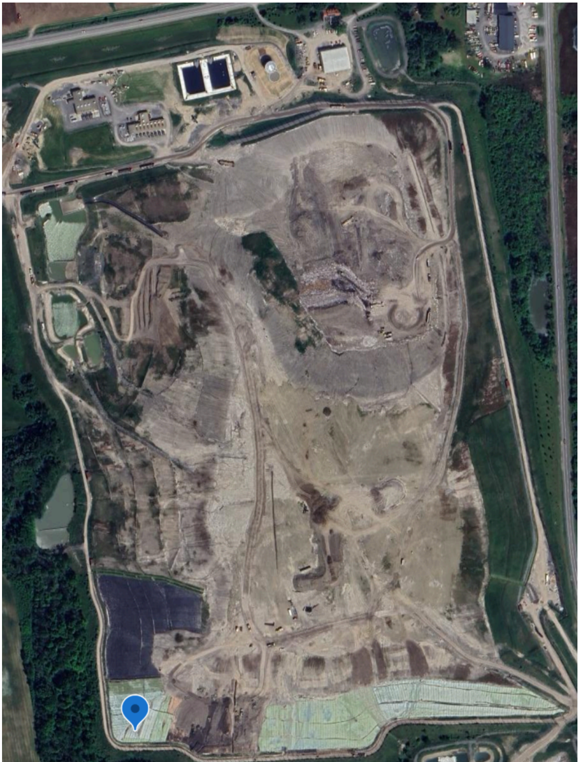
The blue marker shows the location of the November 2023 landslide at the Ontario County Landfill.
