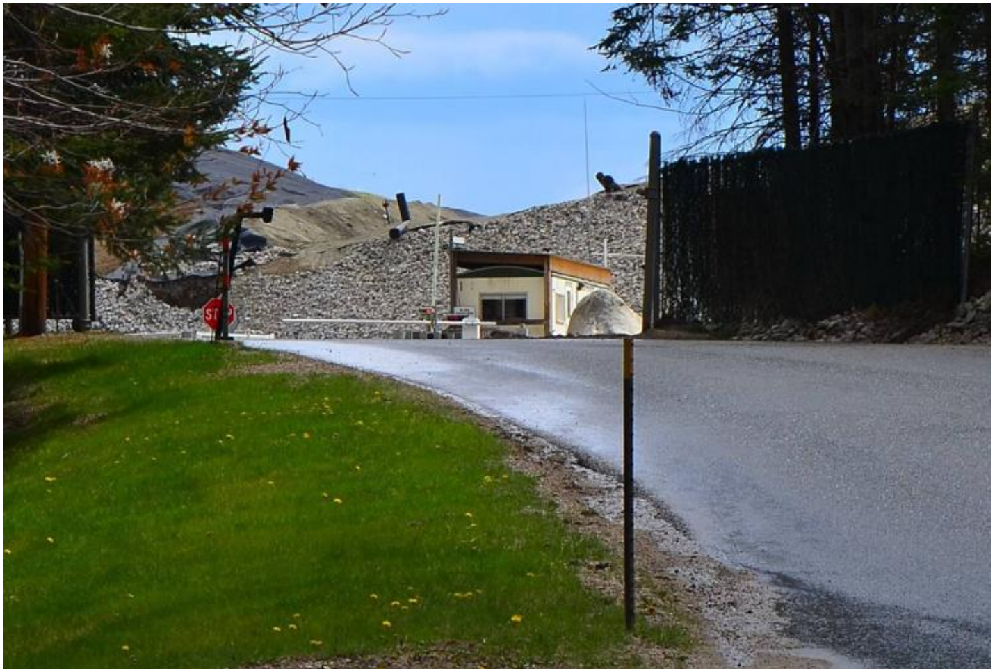
The state has found Casella Waste Systems to be in violation of its operating permit by placing waste outside the permitted vertical limits of its landfill in Bethlehem. (File photo)
