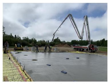
Building continues! The foundation is complete, electrical and plumbing is stubbed in and the slab is being poured in the coming days.
