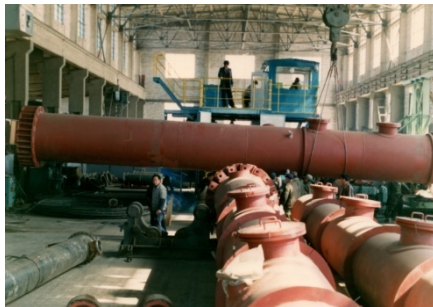
Oil refinery towers
