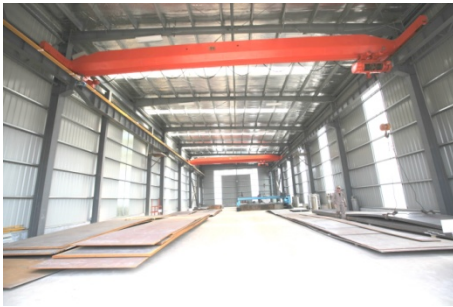
charge make-up area
