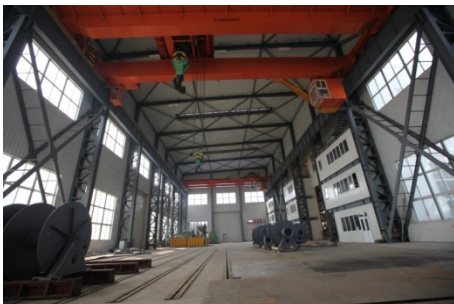
Assembling shop (Crane 100tons )
