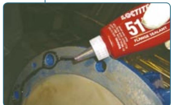
Step #4. Apply Loctite 518 Master Gasket Flange Sealant.
