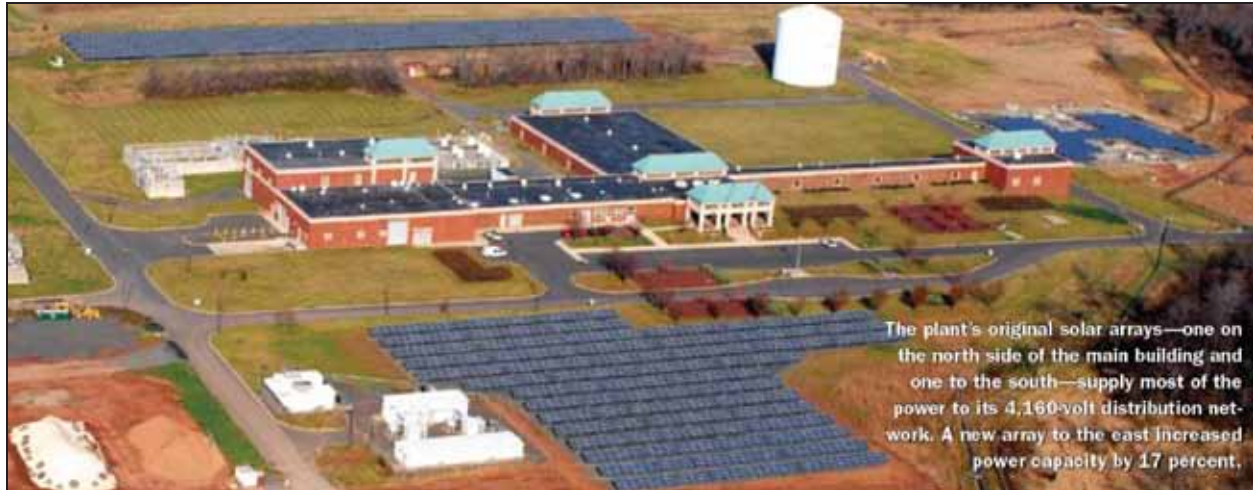
Figure 4.13 Photovoltaic system at NJAW Canal Road WTP
