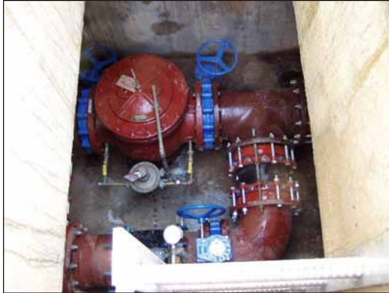
Figure 4.14 Altitude valve at Luzerne Road Tank
