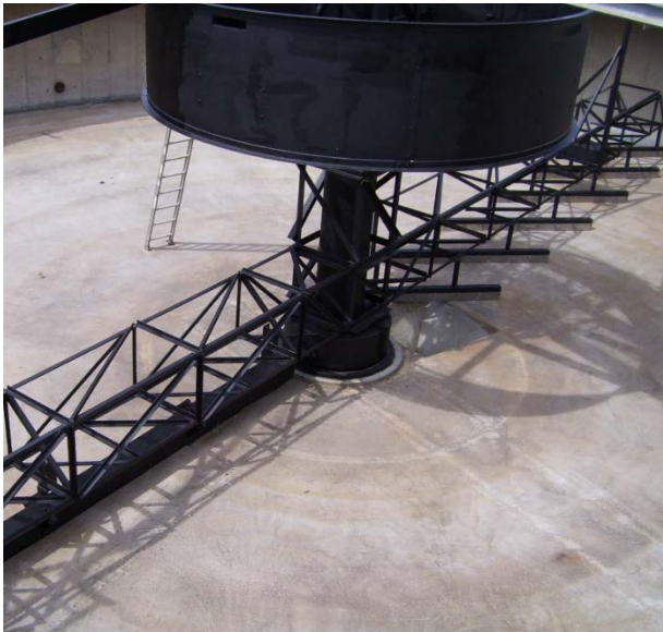
Repair and Replace
