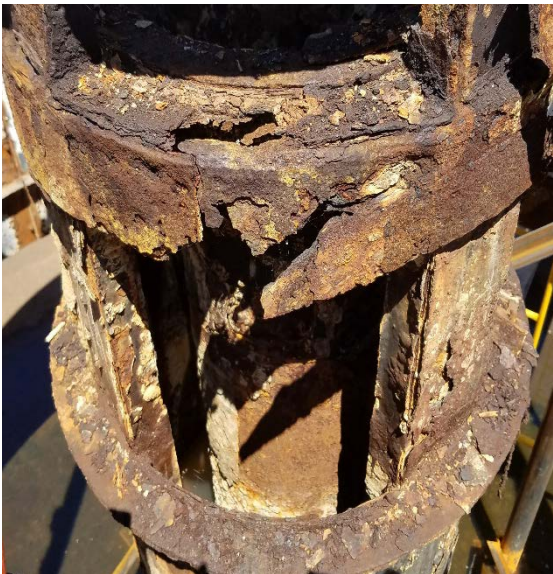
Center Tube Corrosion
