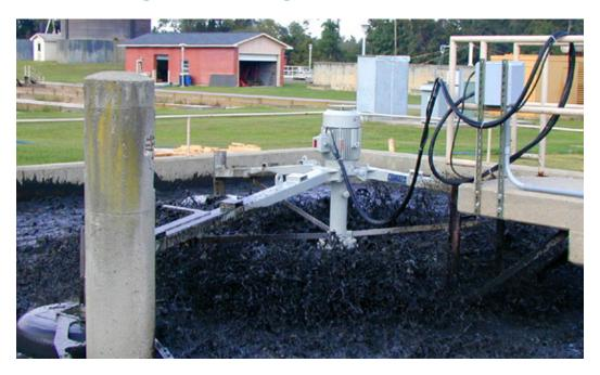
DBS Floating Aerators are ideal for lagoon and aerobic digester applications. The compact design of the NSA floating aerator makes these units easy to assemble and install. All wetted parts such as the aeration rotor, float arm lower link, and float hardware are made from corrosion resistant stainless steel for long life and reliability.
