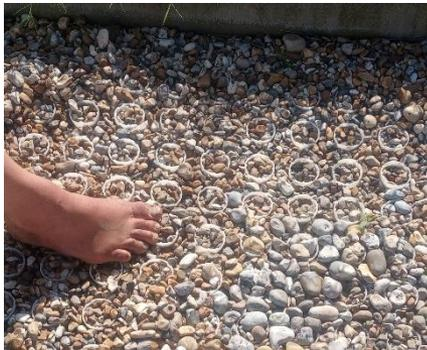
The plastic grid can be seen in this car park application using pea shingle not crushed gravel. An alternative infill with a different mesh is earth and grass.
