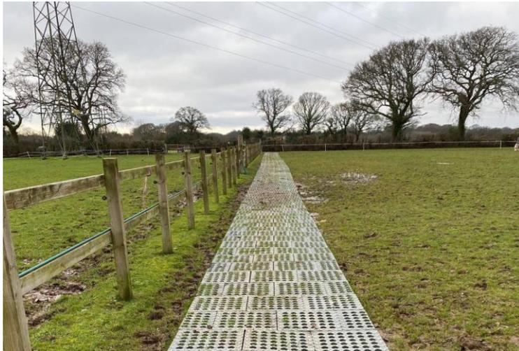
Recycled plastic Ground Stabilising Slabs are used extensively in farmyards and even military training areas. They require no aggregate base and grass is encouraged to grow through the holes
