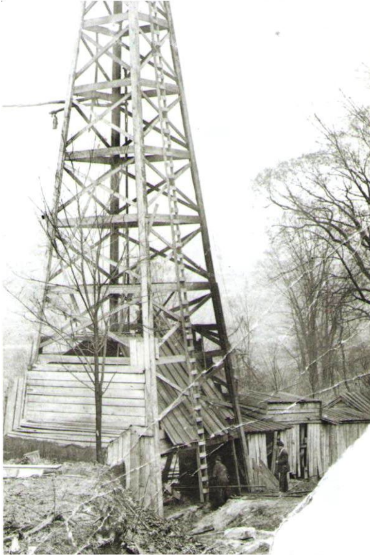
Well site. Photo provided by Linwood Lowden.
