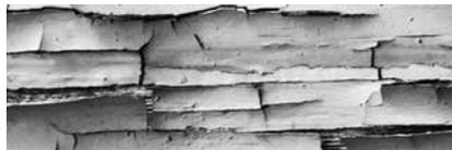
Old varnish that looks cloudy may contain lead. Lead-based paint was often mixed with varnish to give it a deeper, richer color. If the finish is cracked or peeling, old varnish is a **HAZARD** that can cause lead poisoning.
