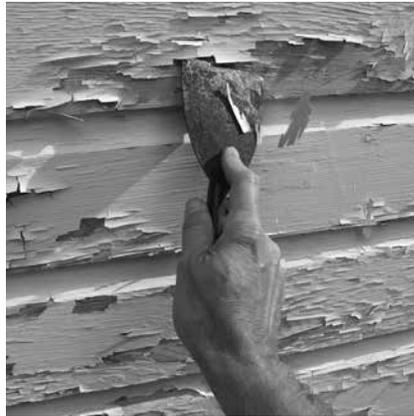
Paint that has an “alligator” cracking pattern or rubs off on your hands (chalks) is usually lead-based paint. Cracked or chalking paint is a **HAZARD** that can cause lead poisoning.
