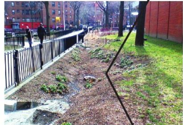
Rain garden system surrounding the Community Center
