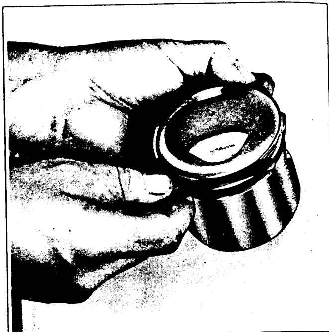
Figure 3C-6. Measuring Ring Side Clearance
