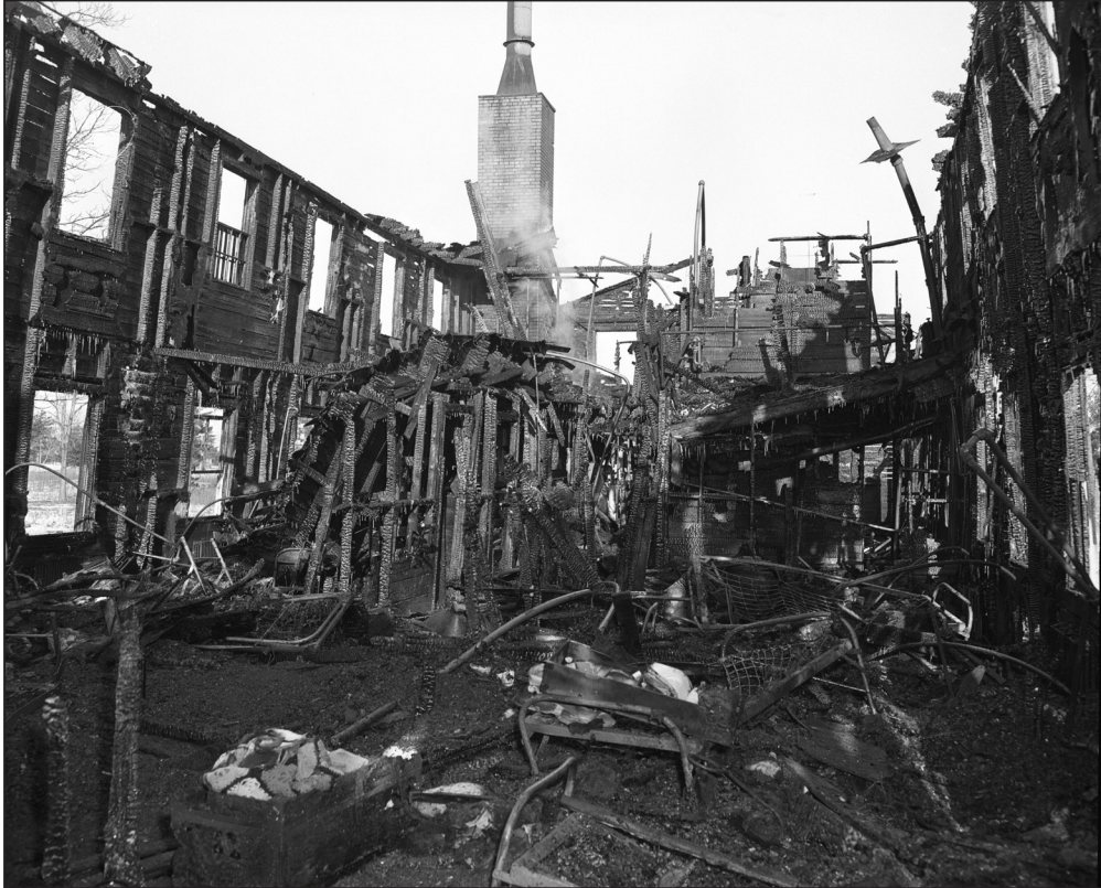
1. Building T-2278 interior ruins (Watertown Daily Times).
