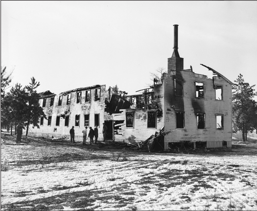
3. Rear and side view of T-2278, note that side exit door appears blocked by fire damage (Watertown Daily Times).
