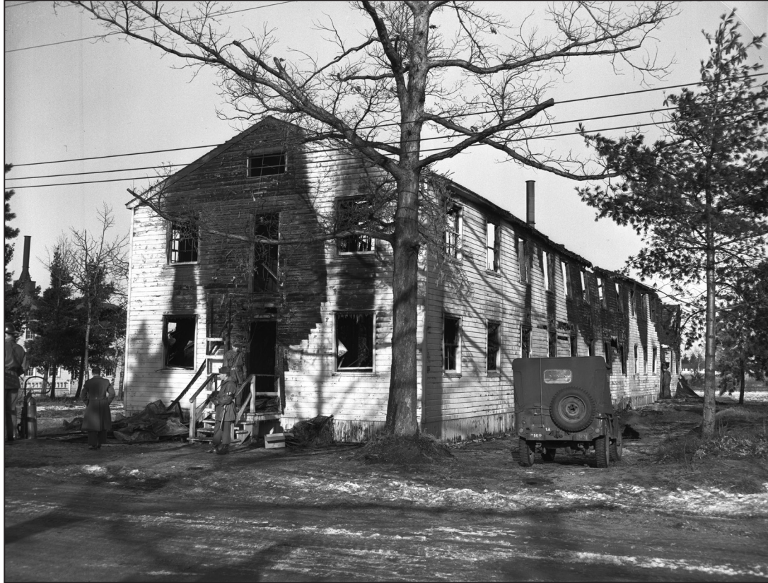
2. Fire investigators inspecting the damage of T-2278 (Watertown Daily Times).
