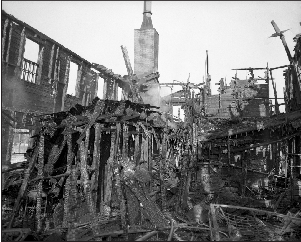
4. Progressing closer to rear of building interior damage (Watertown Daily Times).
