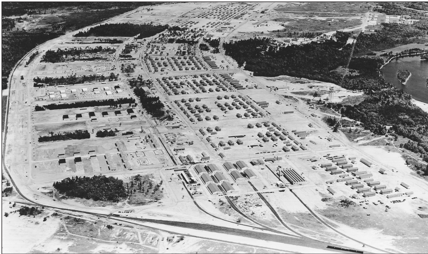
Aerial view of Pine Camp, 1941 (NARA College Park).
