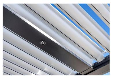
Unlike many other pergola louvers that must remain open during storms, our louvers are engineered to stay closed, providing superior protection and peace of mind. This unique design allows them to handle 40-70 lbs per square foot of snow, depending on the length of the louvers, and withstand winds of up to 120 mph when closed.
