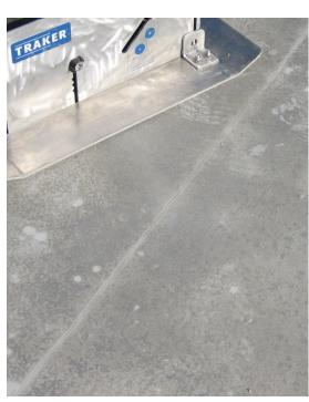
Straight crack develops at Trak-Joint. Photograph taken at age of 3 days.
