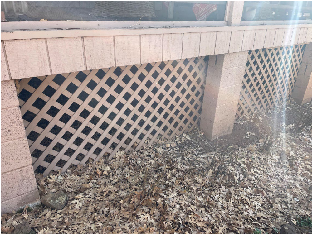
Image 6: To meet FIREWISE standards, consider completely closing under porches and decks, remove pine needles and other forest debris, and use primarily rock and hardscape within the immediate zone (0-5 ft.).
