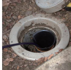
Insert Sleeve in cleanout
