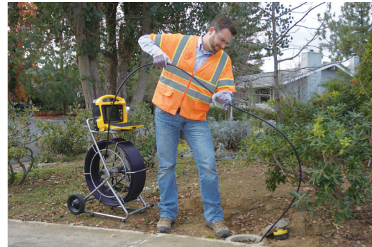
Improper placement and pushing may result in kinking the pushrod.
